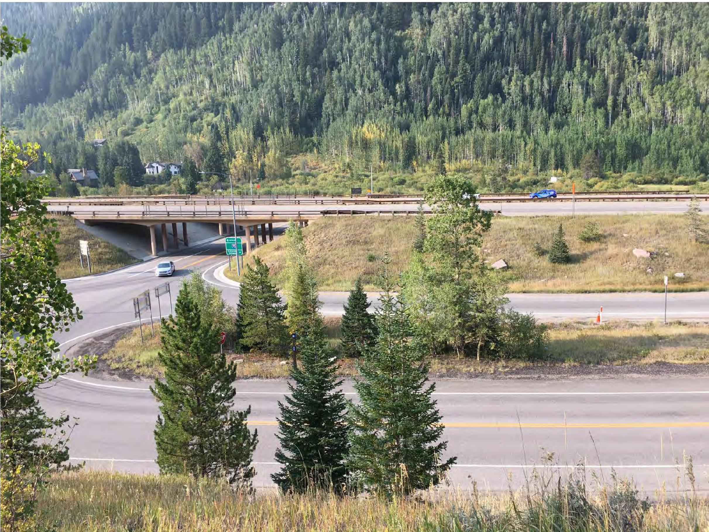
View from property marker (3) to the south
