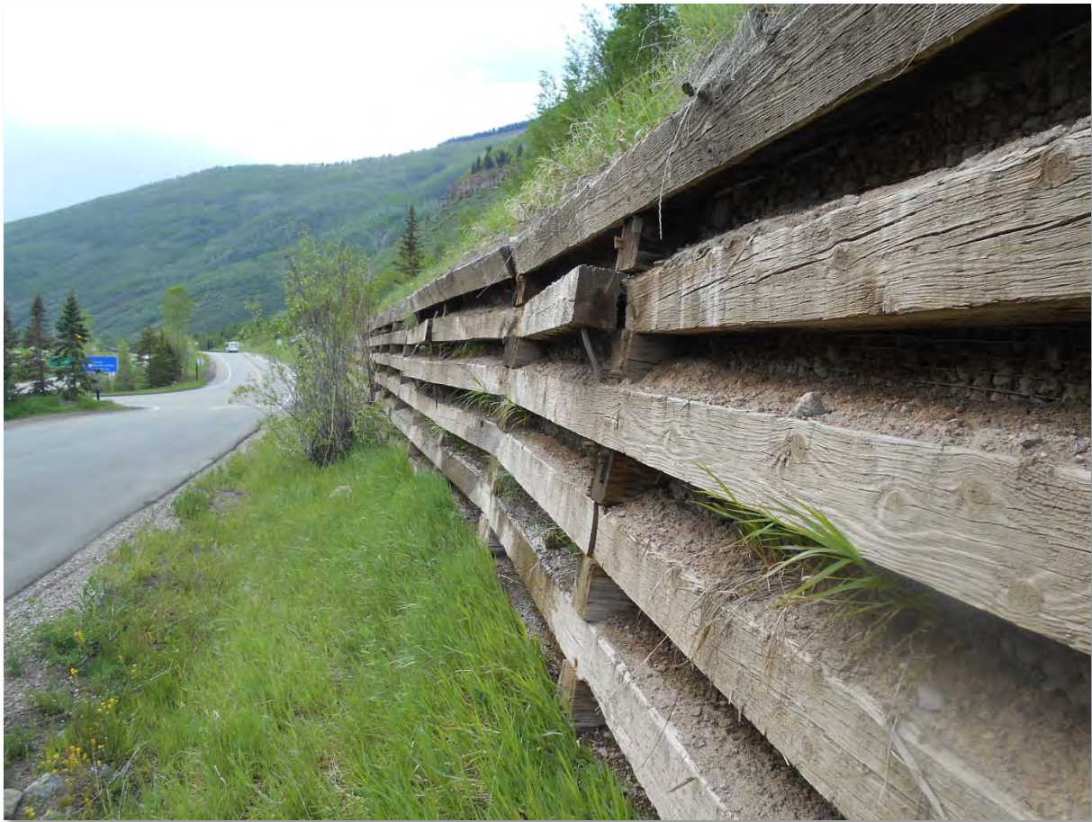
Photograph 3. View of distressed part of the retaining wall along the edge of the site that borders Fall Line Drive. The slope rises steeply upward to the north at the top of the wall. This photograph was taken near the east end of the wall.
