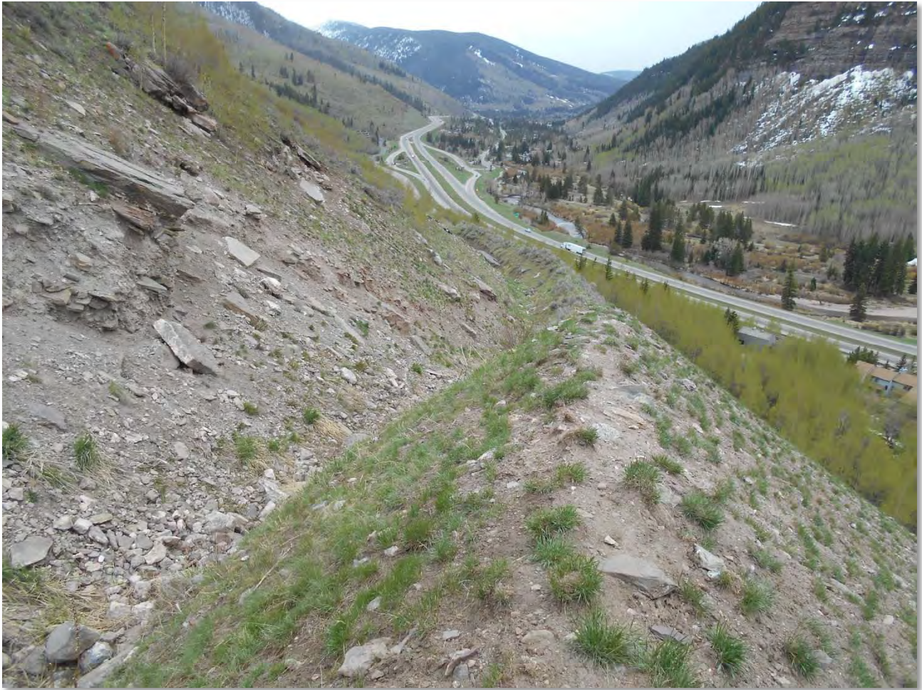
Photograph 11. View of rockfall catchment berm and basin upslope from Booth Falls Subdivision. View looking east toward the project site.
