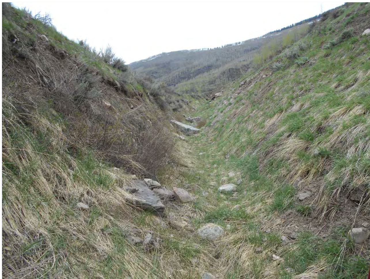
Photograph 10. View of rockfall catchment berm and basin, upslope from Booth Falls Mountain Homes. View looking west toward Booth Creek. The berm is between 10 and 15 feet high, and the ditch is about 20 feet from crest of berm to backslope.
