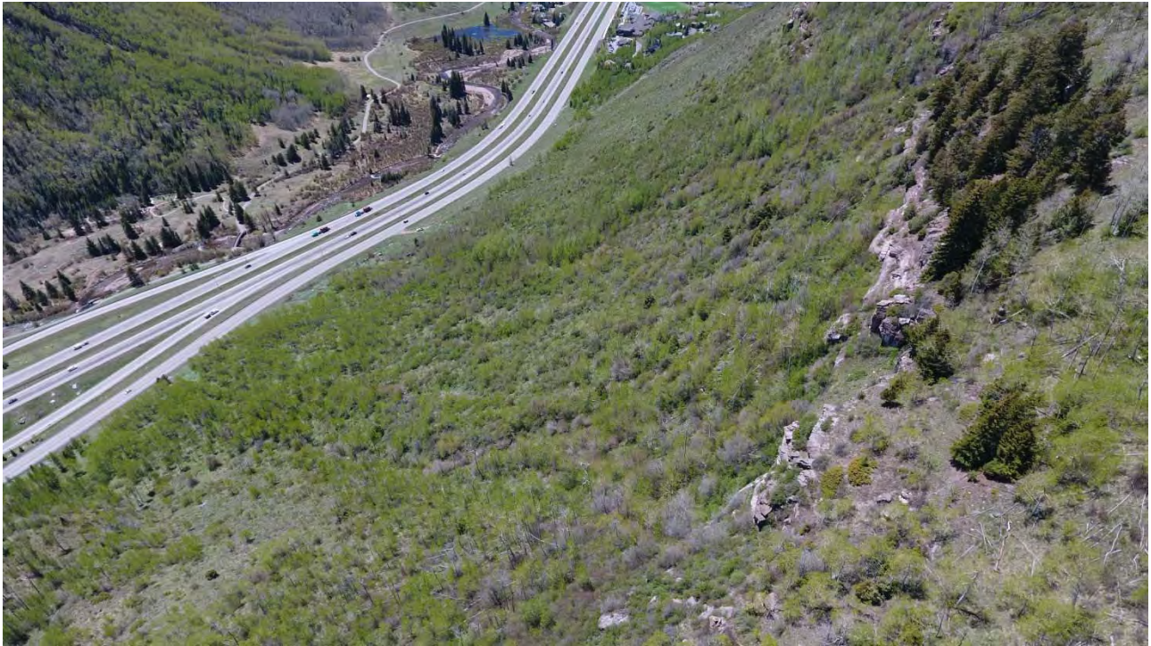
Photograph 15. View looking downslope along the rockfall study section. Notable features include the rock exposures visible at the top of the slope, the steepness of the slope, and the density of the vegetation. Fall Line Drive, I-70, and East Vail are visible in the background.
