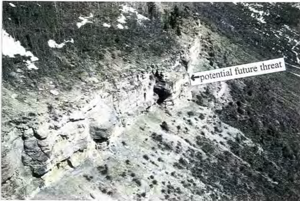
Photo #5. Lower sandstone cliff above district ditch and berm. The CGS will visit this feature this spring and install movement gauges for future monitoring.
