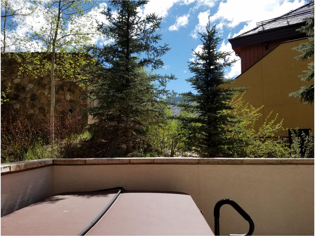
Picture 1 – 1 st Floor Deck
