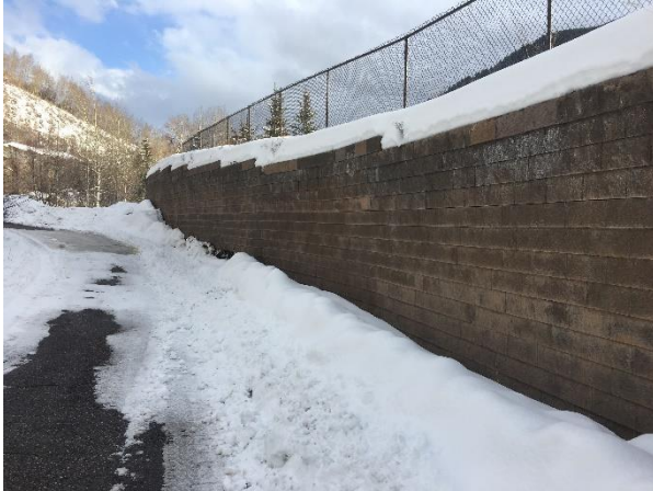
Photograph 1. Existing rockfall impact barrier wall located about 50 feet upslope from existing Booth Falls residences. This system is about 10 feet high, with an additional low capacity, chain link fence at the top. (photo courtesy of Nathan Thompson, GSI)
