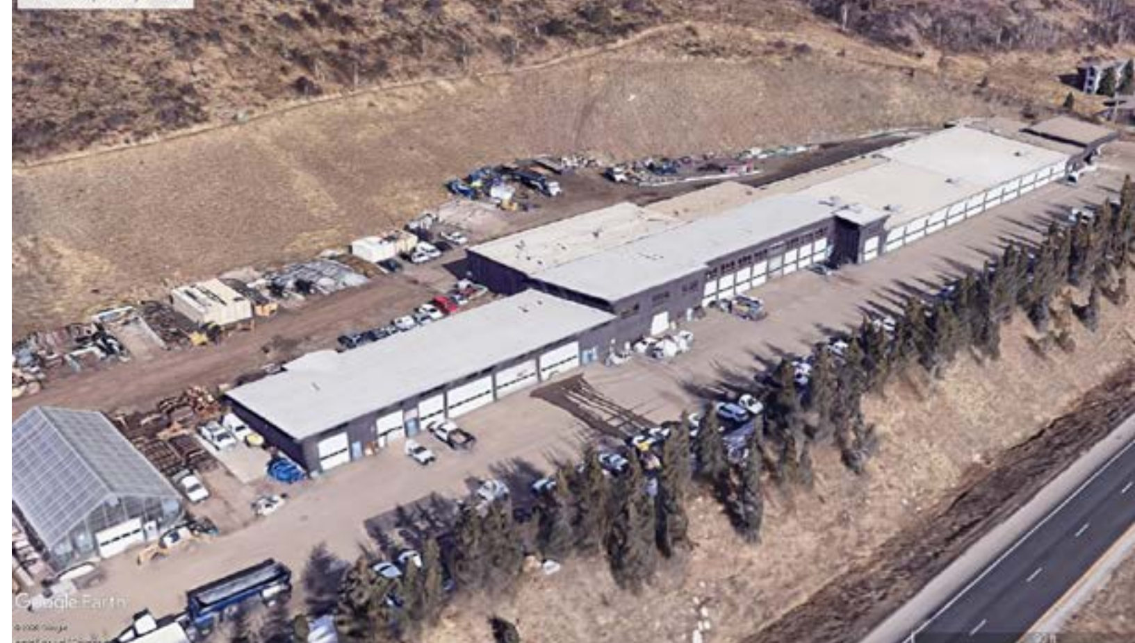
EXISTING SOUTH-WEST SITE IMAGE
