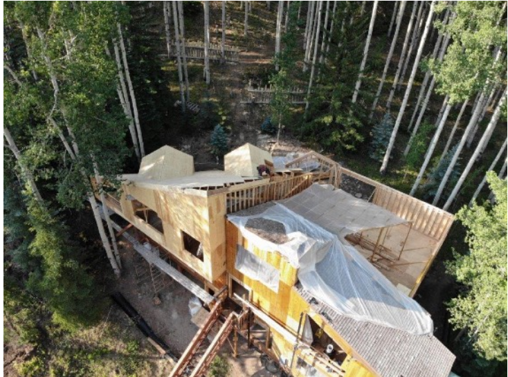
Current construction at 696 Forest Rd.
