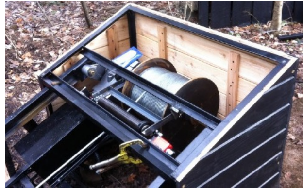
Cable and drum motor system which powers the funicular.
