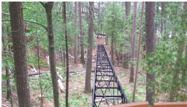
Example of the funicular track proposed and how it can blend with the site.
