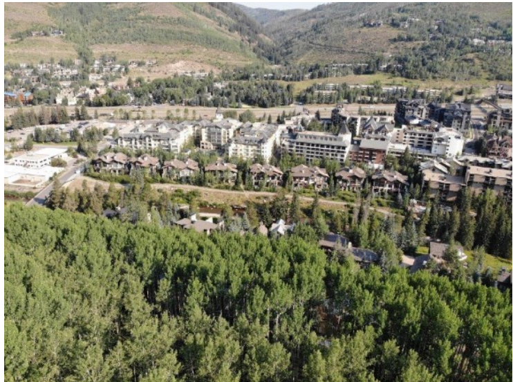
Drone shot of the construction occurring for the recreation facility of 696 Forest Road. The applicant has worked closely with Town staff and DRB to project the existing vegetation.
