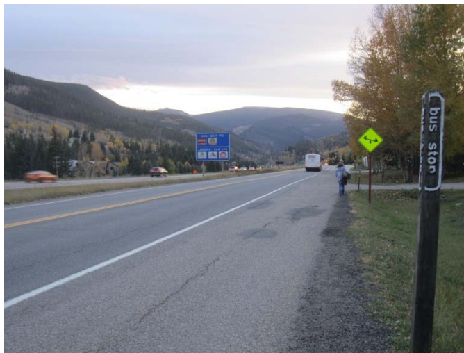
Westbound sight distance at the western site (egress) access
